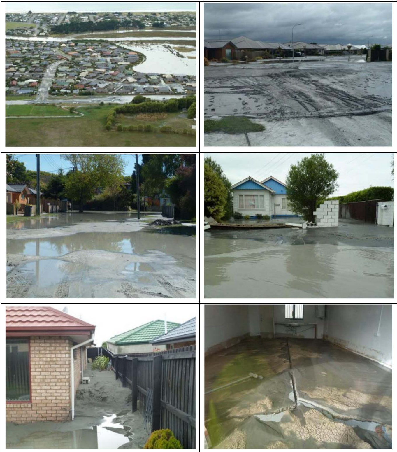
Fig. 1 Observed liquefaction related land damage and residential house damage in Christchurch following the CES [3]
