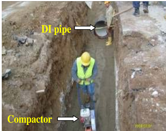
(a) Compacting the DI pipe bed
