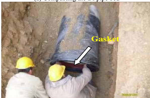
(b) Gasket installment for DI pipe
