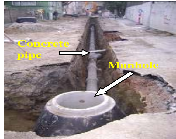
Figure 5. Construction of new sewer system in Denizli
